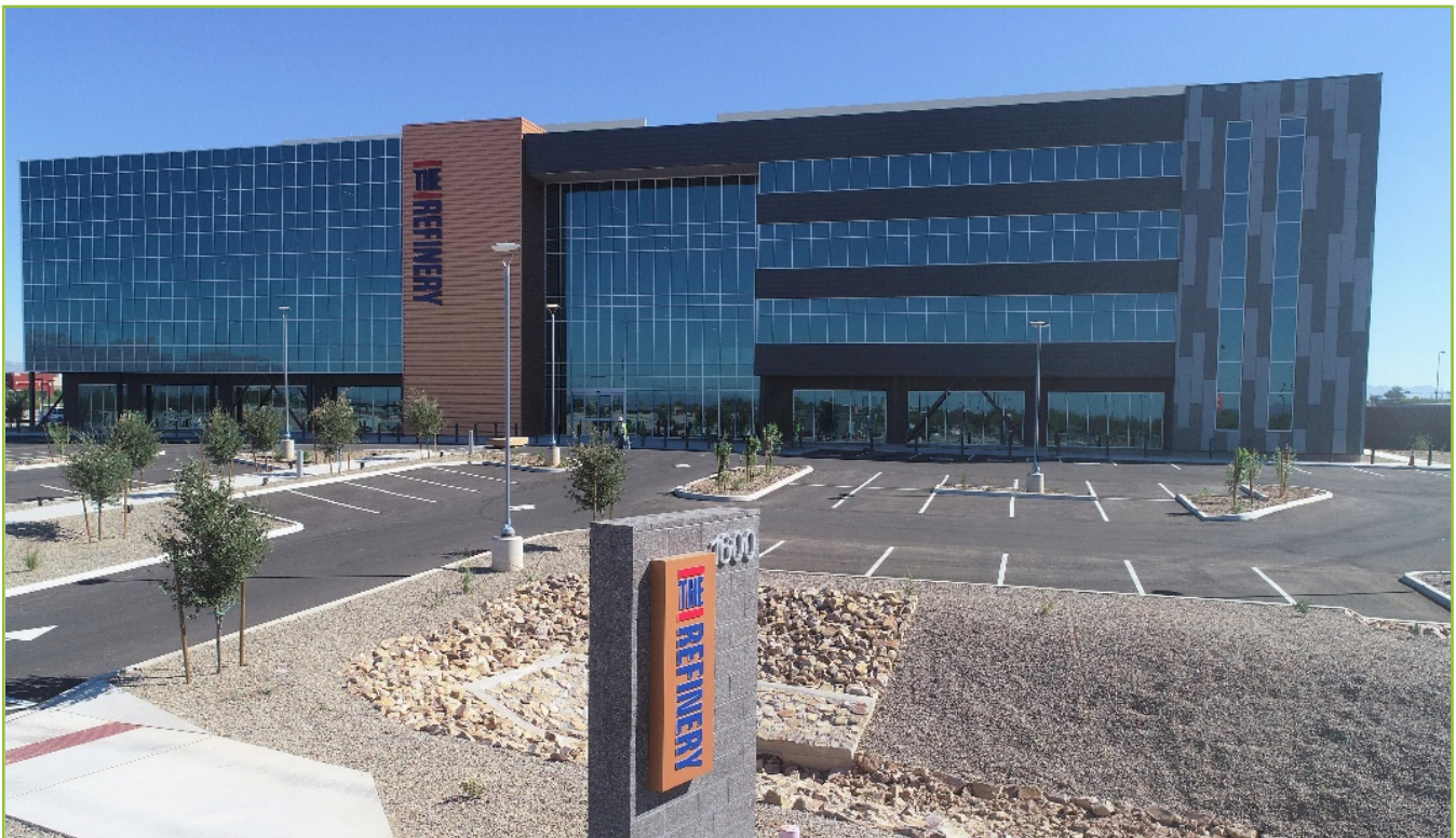
The Refinery (photo courtesy of Core Construction)
