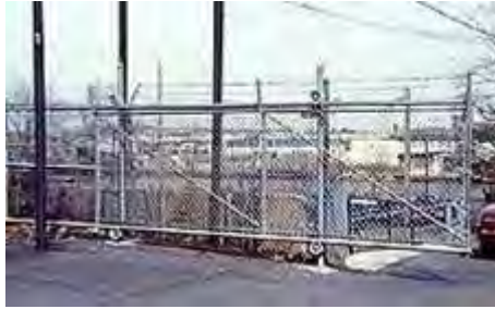
Cantilever slide gates and access control rolling gates providing access to internal parcels from internal service roads inside the Solar Zone.
