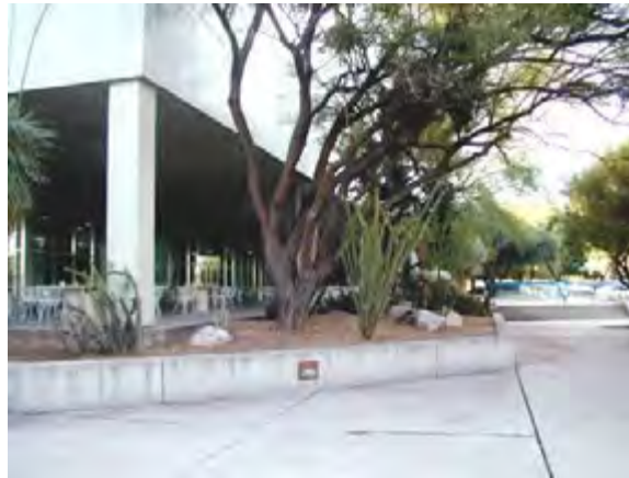
Building cantilever provides shaded seating.
