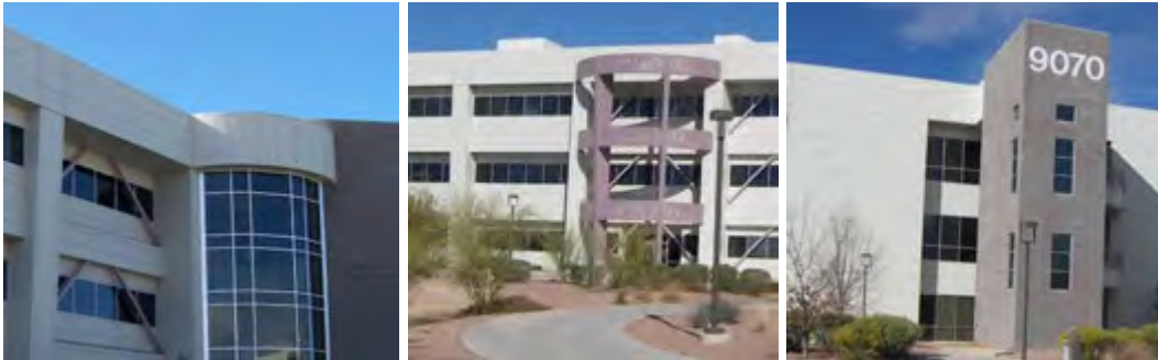
Successful Examples of Utilization of Window Panels, Reveals, Recesses, Projections and Decorative Structures to Segment and Articulate Exterior Wall Surface
