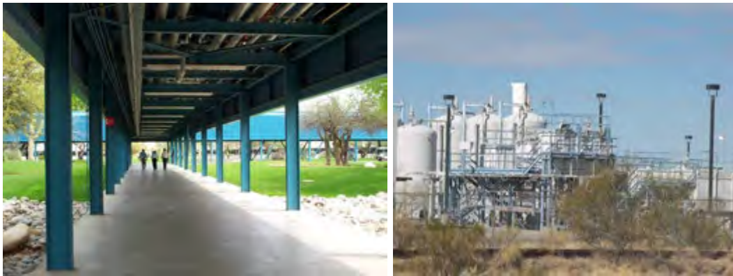
UA Tech Park Utilities Spine, Industrial Waste Water Treatment Facility and Rail Road Spur
