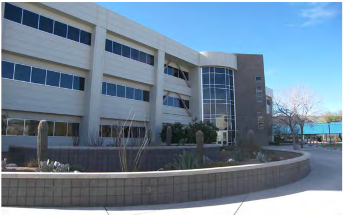
Building 9070 – Attractive High-Tech Architecture
