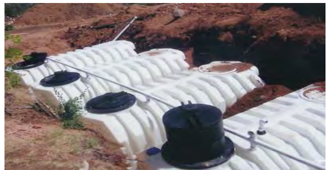
Active Water Harvesting Techniques Above-ground Tanks and Below-ground Cisterns
